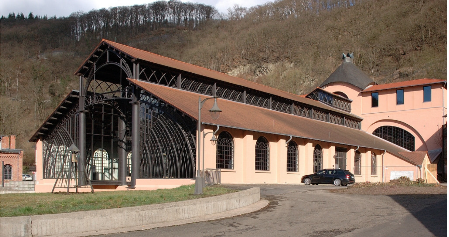
The foundry hall from 1830/1845 with the old warehouse from ca. 1830 on the right and the factory hall from 1909 on the left. Photo: Florian Fichtner 2019.
