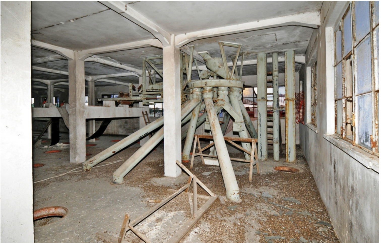
One of the rotating distributor units for filling cells in the Silos, with the characteristic Hennebique reinforced concrete structure.
