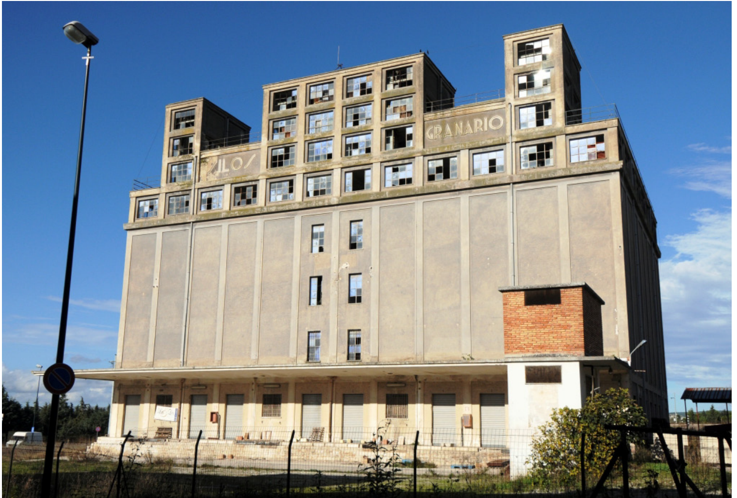
The current condition of the Grande Silos Granario, Gravina.
