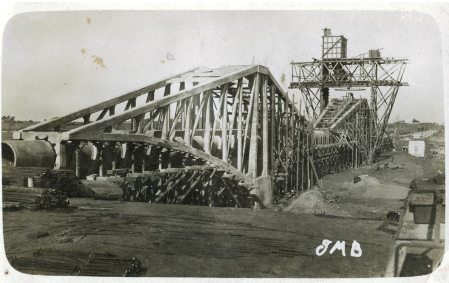
Construction of the Ovoid Sewer Aqueduct over the Barwon River; Breakwater; c.1915, photo; J M B, Geelong Heritage Centre Archives , Australia GRS 2009/419
