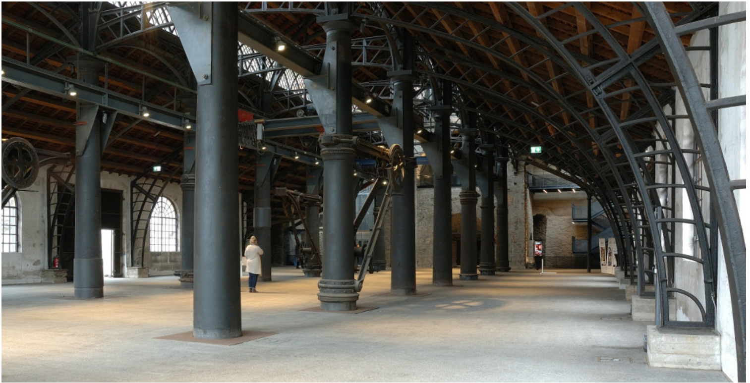
Inside the foundry hall with the iron slewing cranes mounted with ball bearings on the central columns and the blast furnace at the back. Photo: Florian Fichtner 2019.
